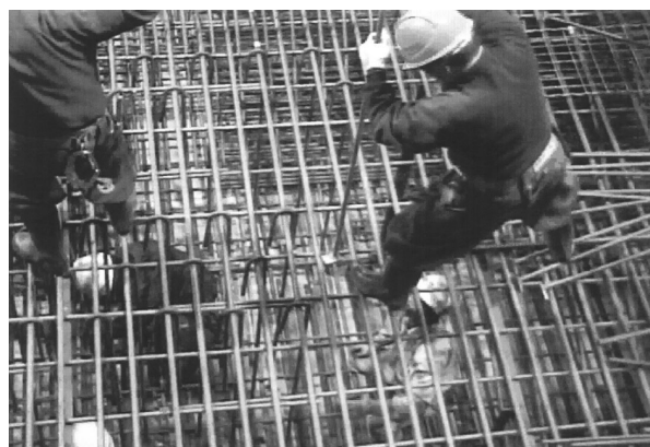
(b)底版の施工
